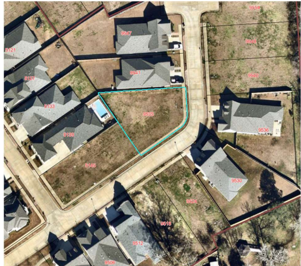
Figure 1: Aerial view of the Site and its surrounding
