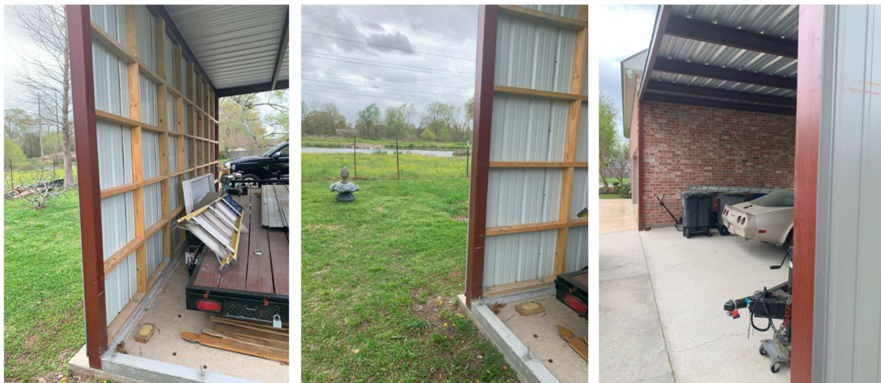
Figure 3: Photos of the addition at its current condition, submitted by applicant
