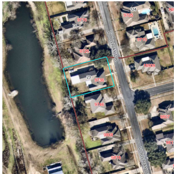
Figure 1: Aerial view of the Site and its surrounding
