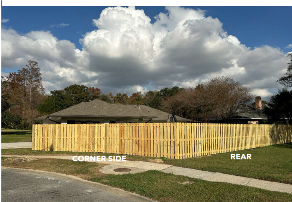
Figure 5: Photo 2 of the constructed fence in the corner side yard, 12/18/2024.
