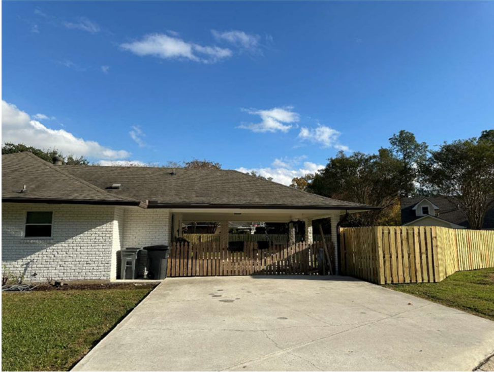
Figure 4: Photo 1 of the constructed fence in the corner side yard, 12/18/2024.
