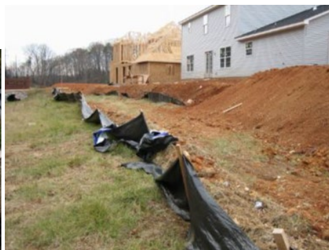
Silt Fence Fails
