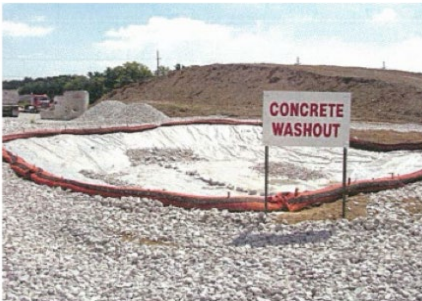
Concrete washouts areas are designated locations within a construction site that are either a prefabricated unit or a designed measure that is constructed to contain concrete washout. Concrete washout systems are typically used to contain washout water when chutes and hoppers are rinsed after delivery.
