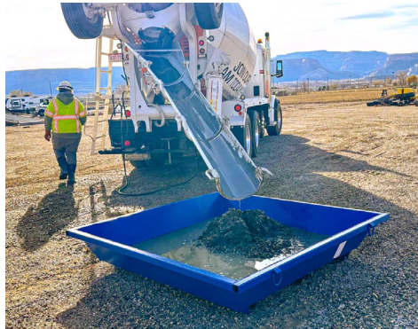
Concrete washouts areas are designated locations within a construction site that are either a prefabricated unit or a designed measure that is constructed to contain concrete washout. Concrete washout systems are typically used to contain washout water when chutes and hoppers are rinsed after delivery.
