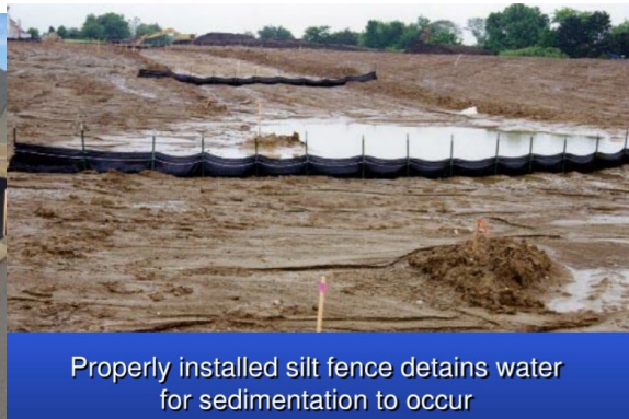
Properly Installed Silt Fences
