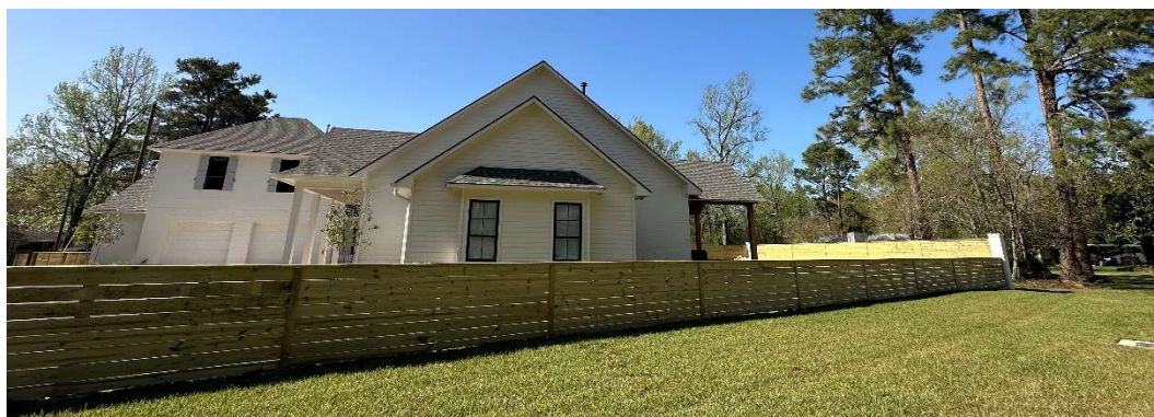
Figure 2: Current fence situation. Photo taken by staff planner during site visit on 3/21/2025.
