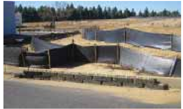
Figure 25: Sediment control BMP - silt fencing
