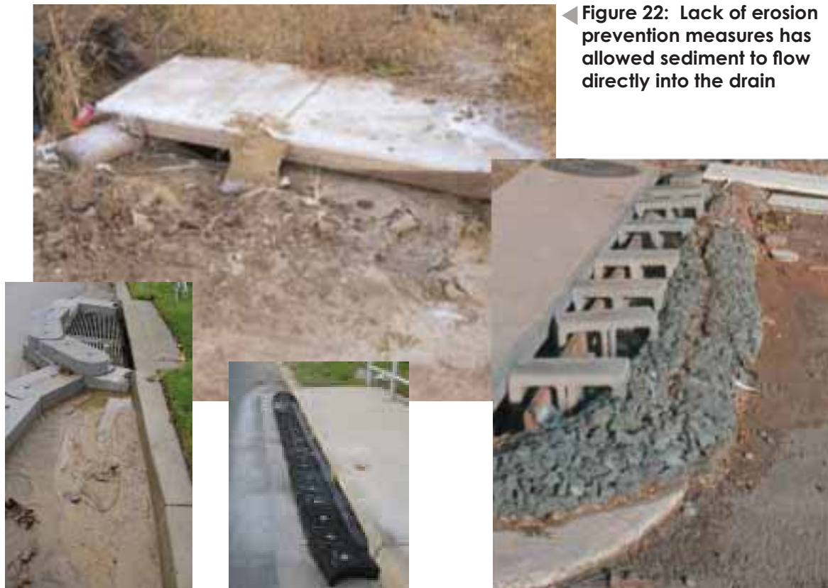
▲ Figure 23: Drain inlet protection employed to prevent sediment from entering the storm drain system
