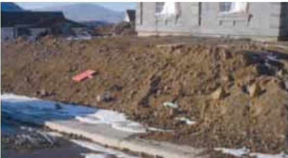
Figure 28: Sediment from unstabilized bank has washed out onto the sidewalk
