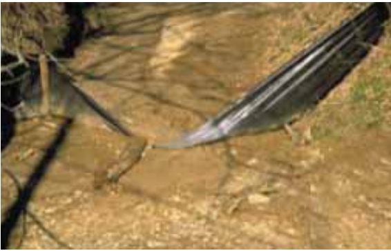
Figure 27: Erosion control BMPs must be maintained throughout construction to ensure that they are functioning properly
