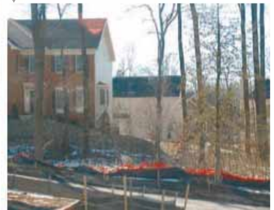
Figure 26: Construction with erosion prevention measures
