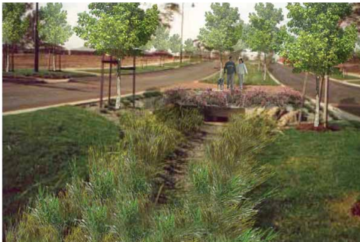
Figure 13: Roadway with a biofiltration median
