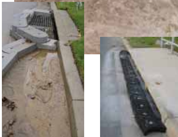
▲ Figure 23: Drain inlet protection employed to prevent sediment from entering the storm drain system
